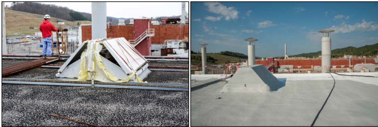
Fig. 2. Before and After Pictures of the Alpha 5 Roofing Project.
