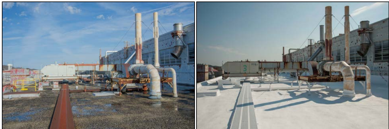
Fig. 3. Before and After Pictures of the Beta 4 Roofing Project.
