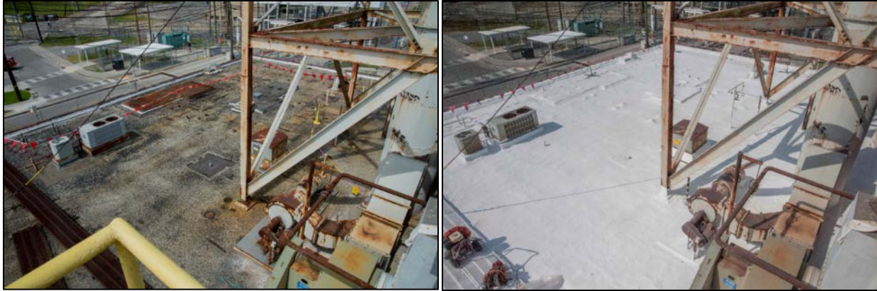
Fig. 4. Before and After Pictures of the Building 9206 Roofing Project.
