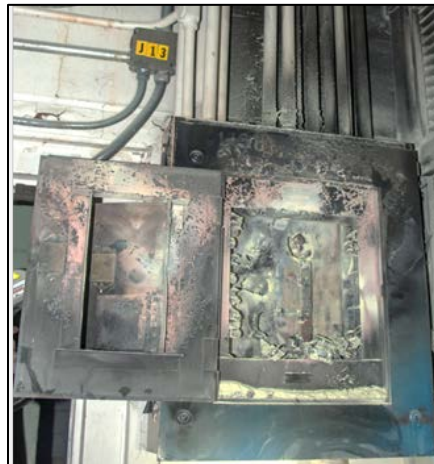
Fig. 7. Example of Obsolete “Burned” Distribution Panel.
