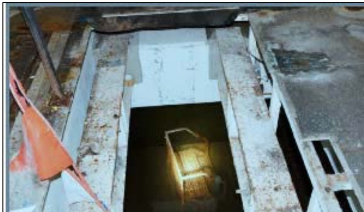
Fig. 5. Flooded Wind Tunnel in Alpha 5.
